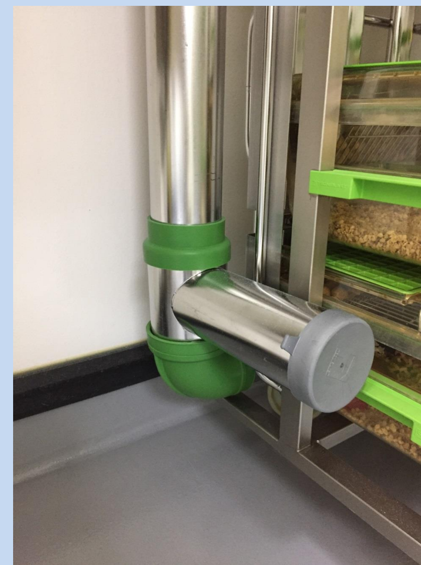
Figure 3. Prototype plenum attachment connected to the exhaust plenum.
